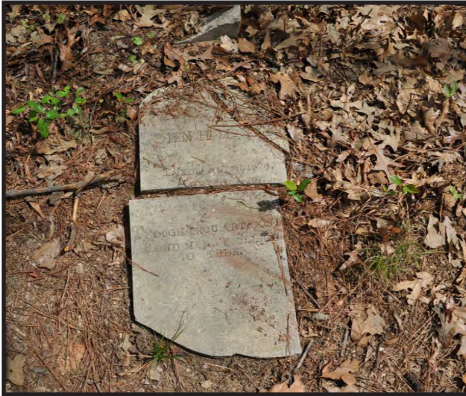
Figure 71. Broken Concrete Marker
