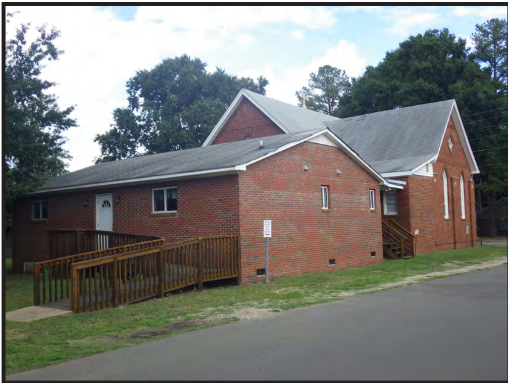
Figure 42. View of Additions Looking Northeast
