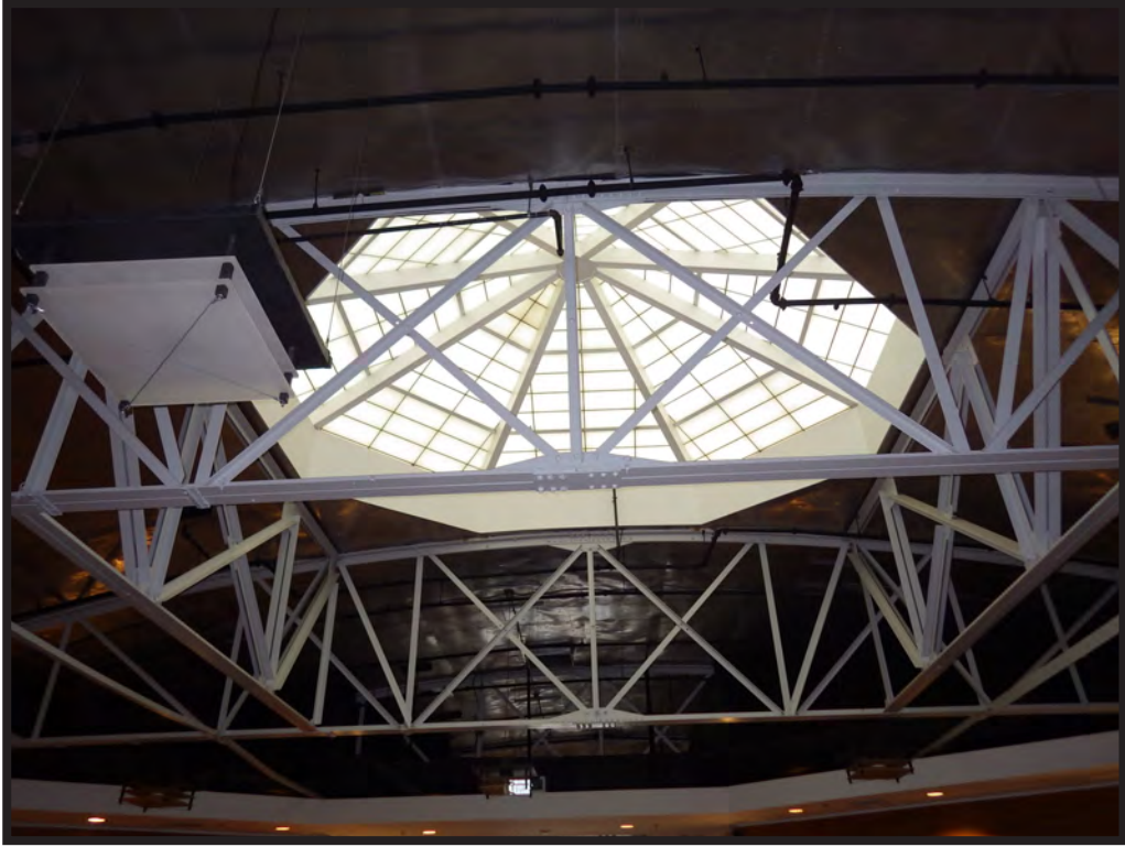
Figure 14. Interior, Steel Bow Trusses
