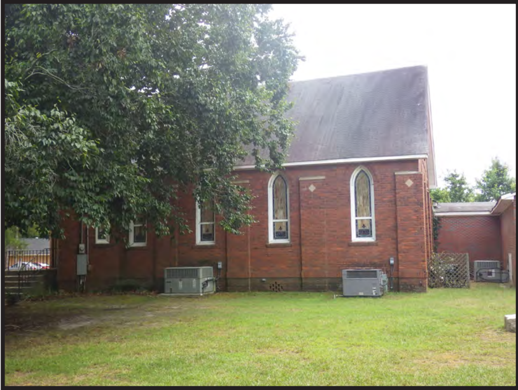
Figure 45. North Side Showing Buttresses with Concrete Caps
