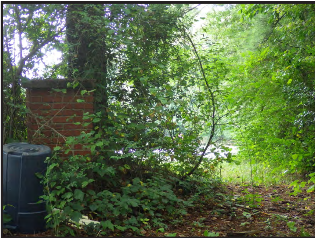
Figure 68. Gate Pillar at Northeast Corner
