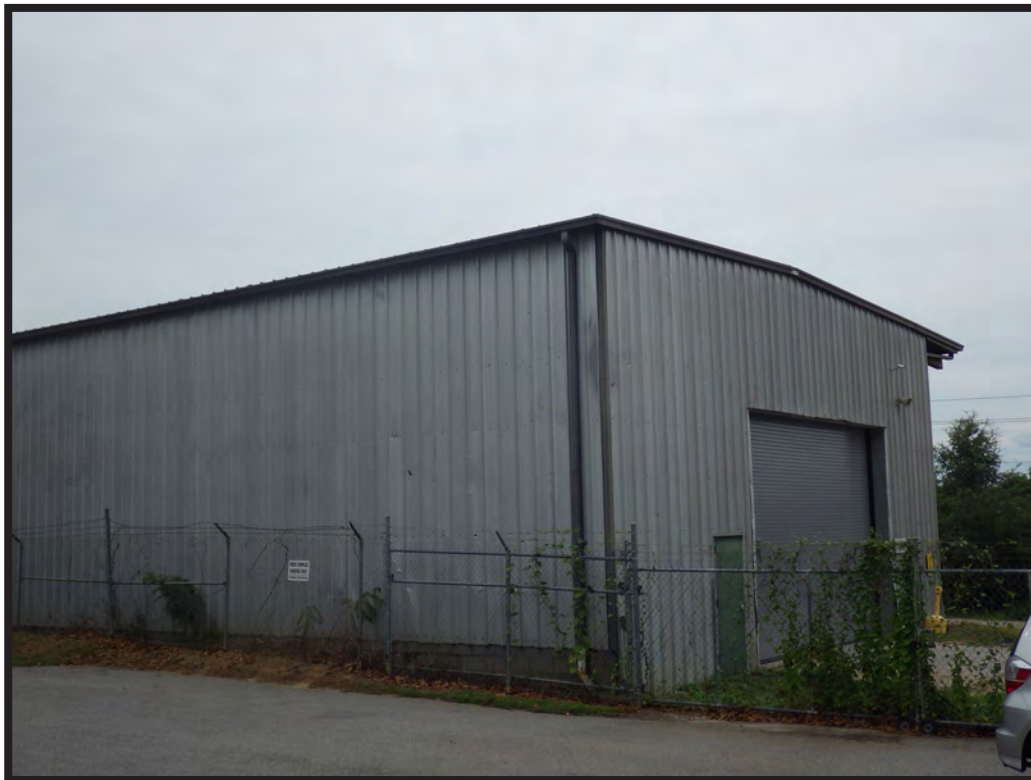
Figure 101. Warehouse #2, Southeast Corner
