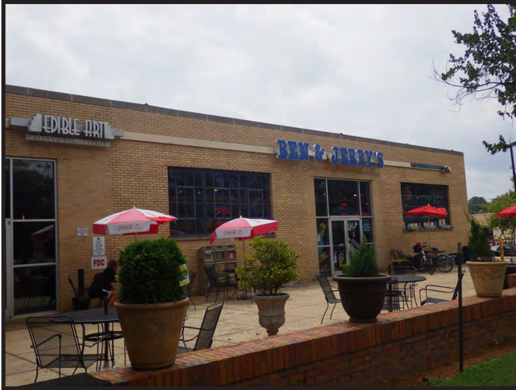
Figure 6. Royal Baking Company North Side, Fenestration Changes on North Wall of West Production Bay
