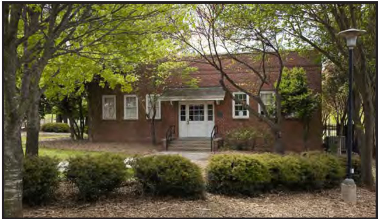
Figure 20. Agriculture Building, North Side
