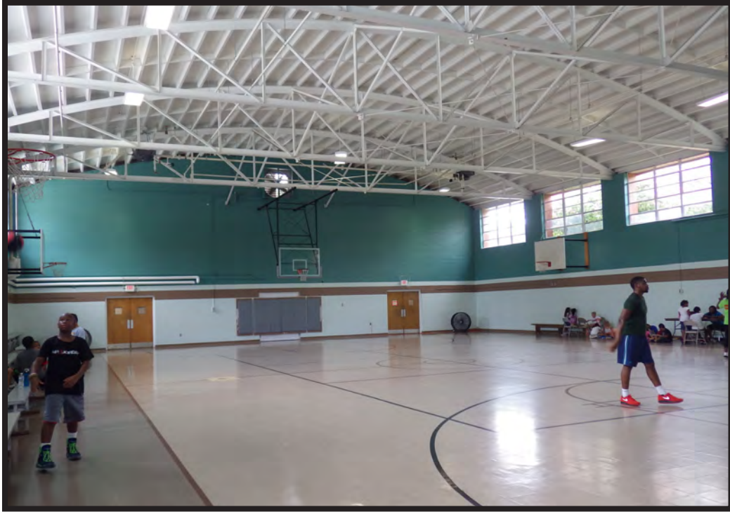
Figure 36. Gym Interior, Looking West
