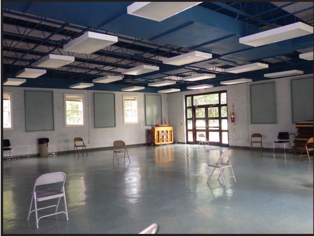
Figure 29. Interior of Addition, Looking Southeast
