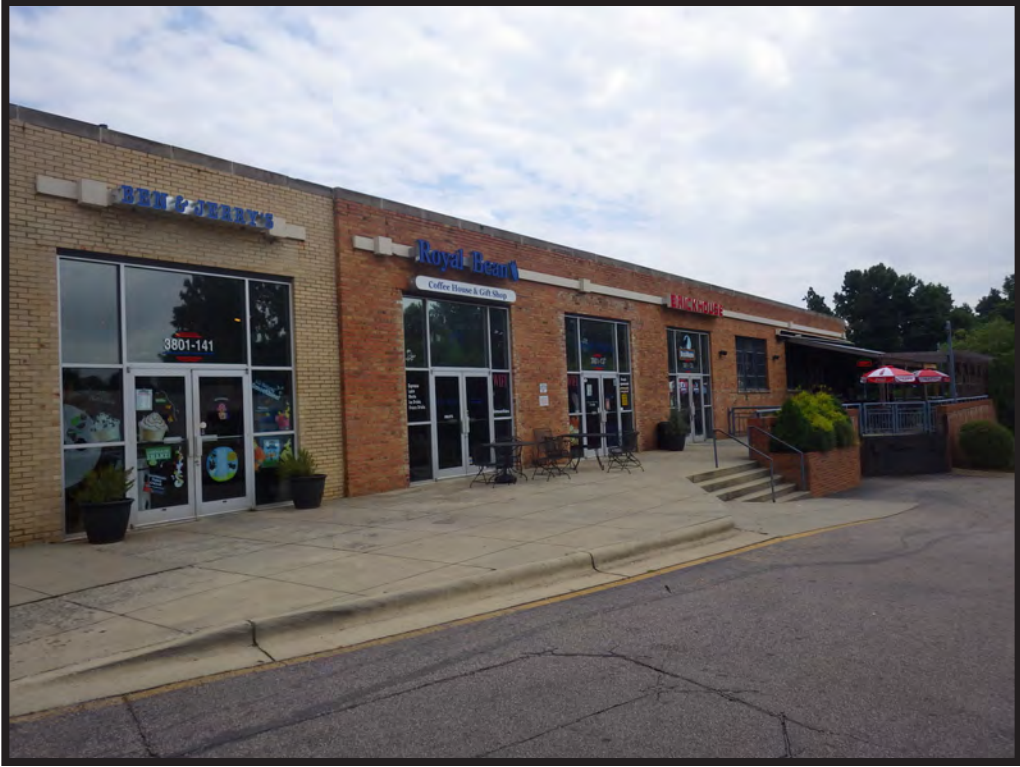
Figure 8. Royal Baking Company, West Side, Fenestration Changes to West Wall
