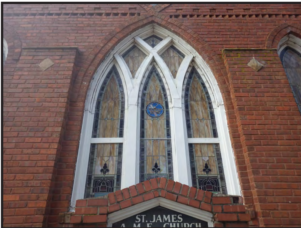
Figure 44. Detail of Triple Center Window on Façade
