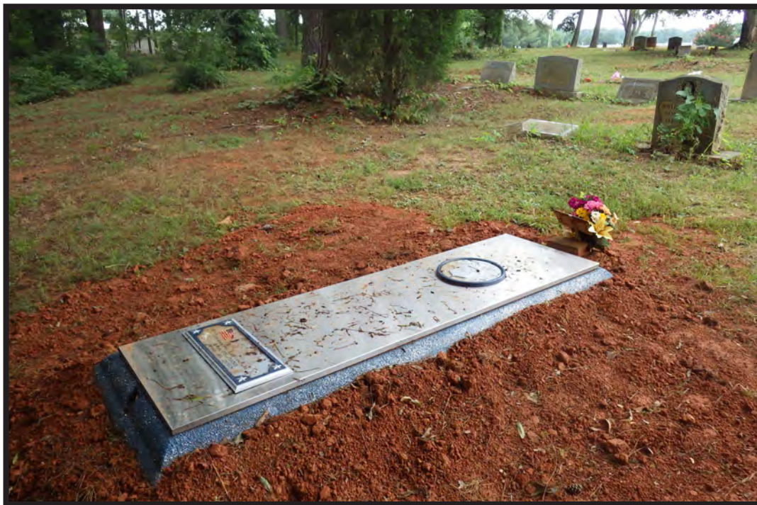
Figure 78. Homemade Blue Concrete Ledger of Rudolph Loftin, Jr. Note reflective material in concrete mix and sheet metal top.
