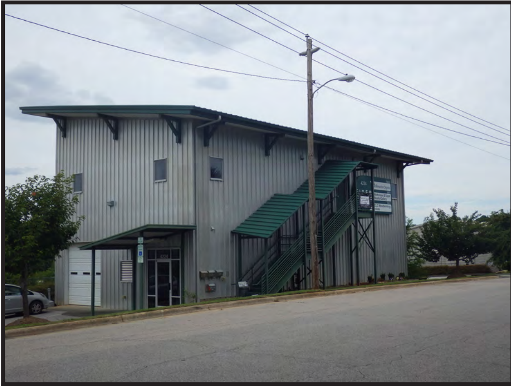
Figure 100. Nicholson and Sayer Studio, Southwest Corner
