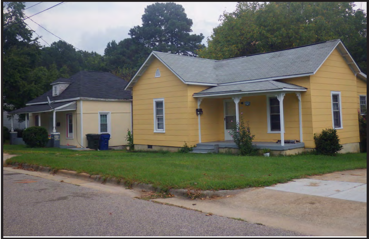
Figure 85. Dwellings on South Side of Woods Place
