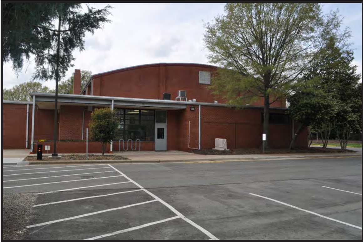
Figure 30. Front (East) Side
