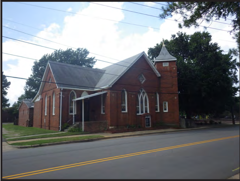
Figure 47. Oblique of Front View Looking Northwest
