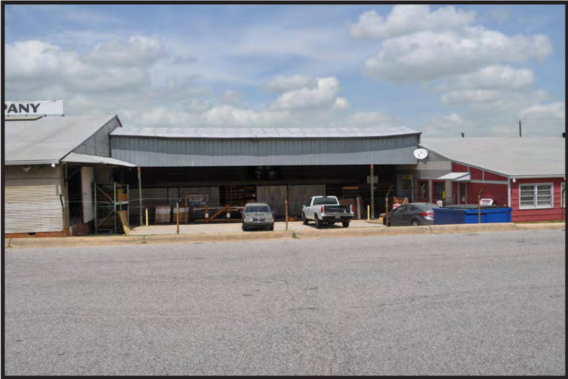
Figure 92. Main Retail Saw Shed, South Side
