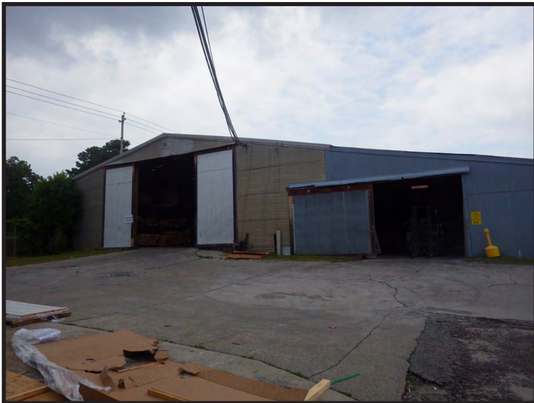
Figure 99. Lumber Storage Warehouse #1, East Side
