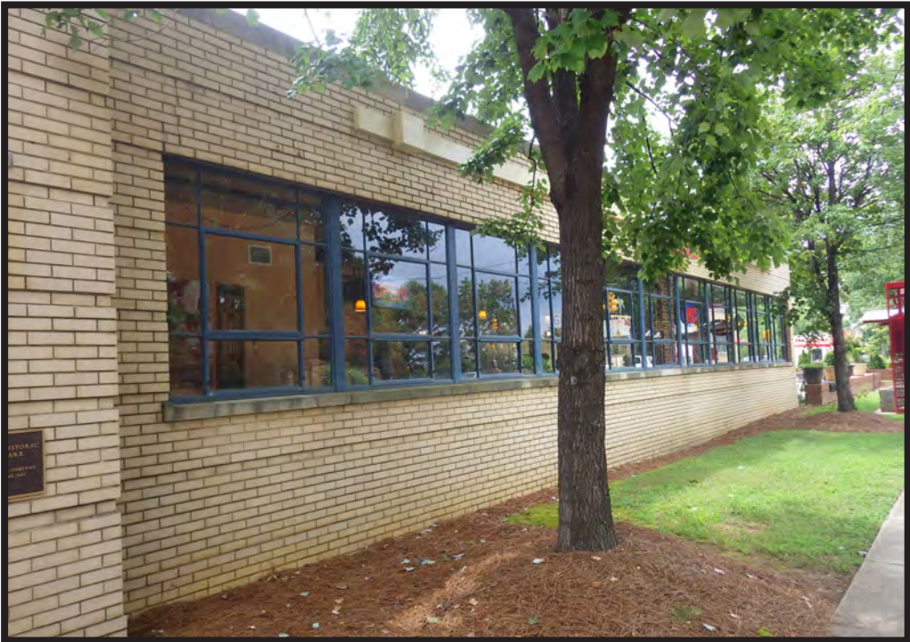
Figure 5. Royal Baking Company, North Side, Original Windows on West Office Wing
