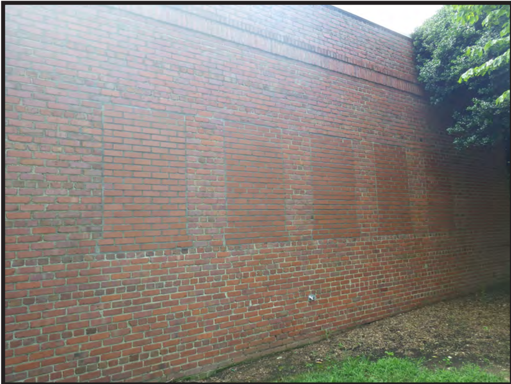
Figure 24. Filled Windows on East Wall of 1928 Section
