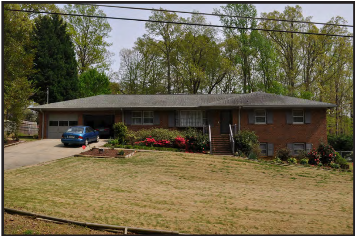
Figure 123. Hipped-Roof Ranch at 1237 Kingston Ridge Road
