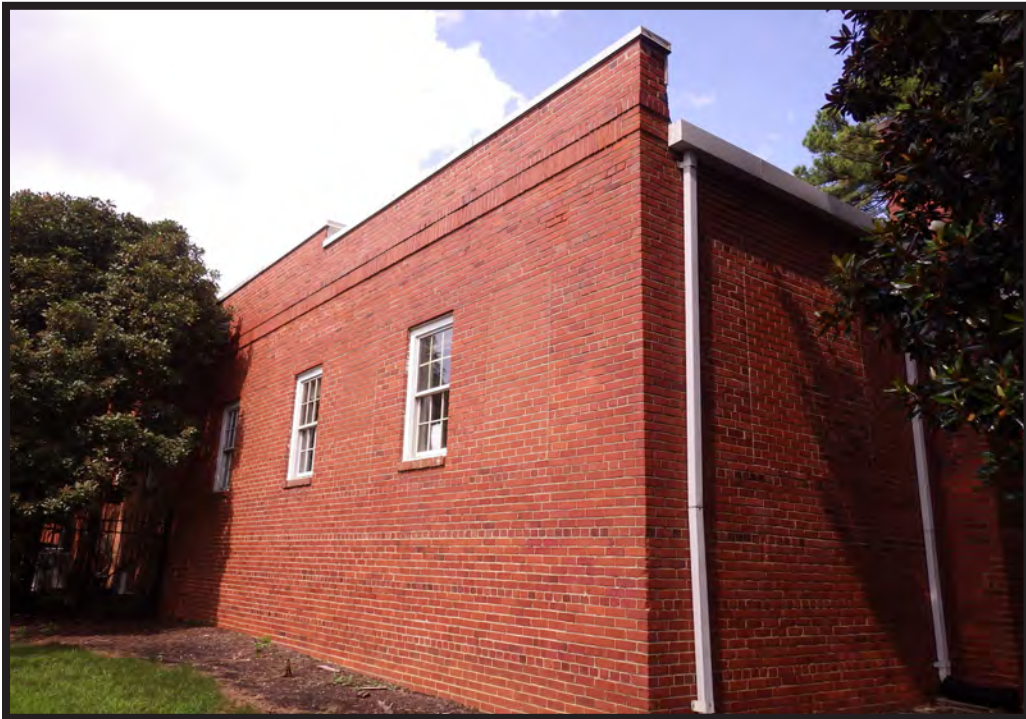
Figure 22. Southwest Corner of Circa 1950 Addition Showing Intersection West Side Parapet Wall
