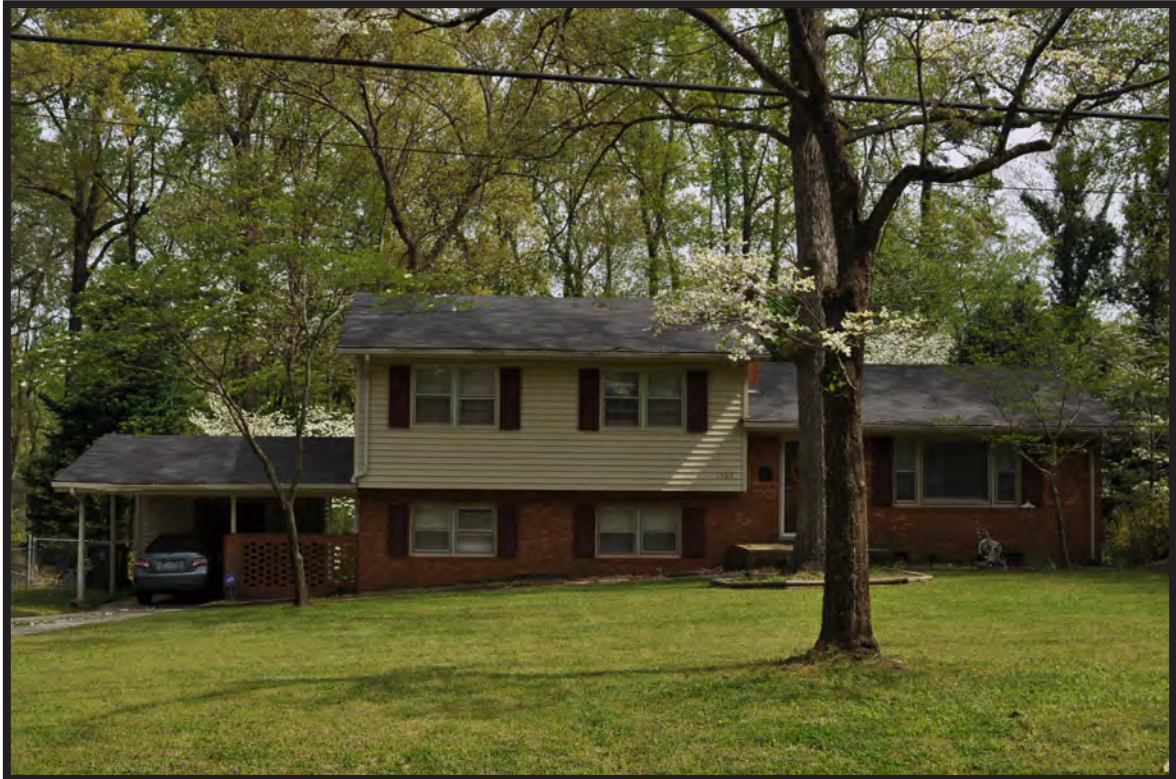
Figure 125. Split Level at 1307 Kingston Ridge Road
