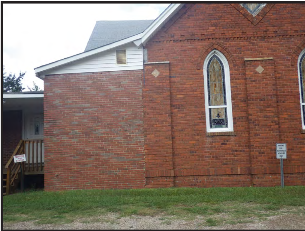
Figure 48. South Side, View of Connection of Shed Addition and 1923 Church
