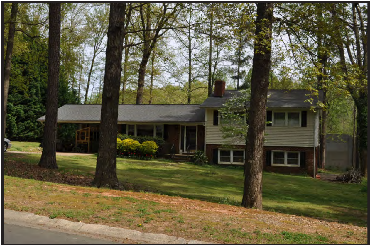
Figure 127. Typical Example of Vinyl Siding and Windows
