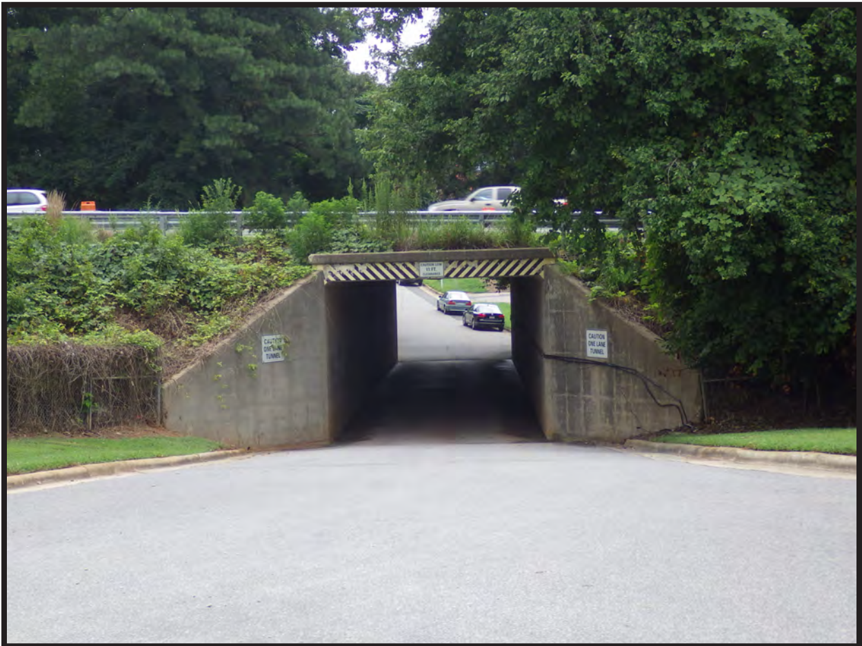
Figure 65. Tunnel Under I-440
