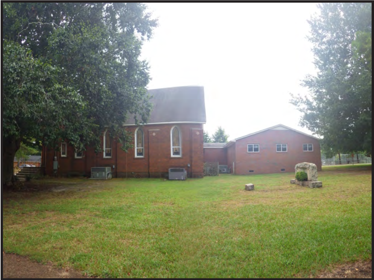
Figure 49. View of North Side Showing Gabled Addition and Hyphen
