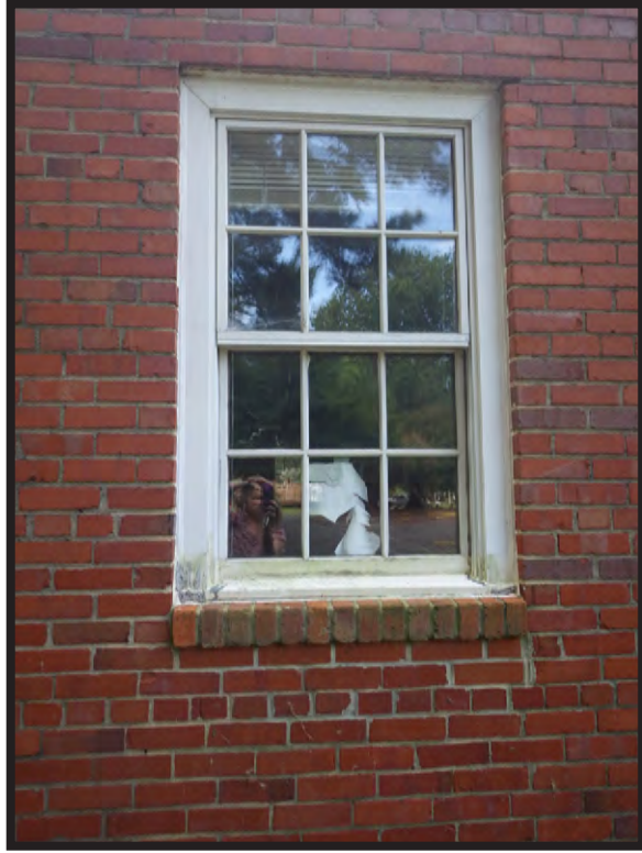
Figure 25. Replacement Windows on East Wall of Circa 1950 Section
