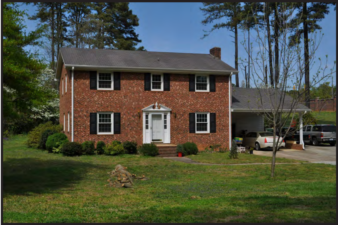
Figure 124. Two-Story House at 1006 Fairlane Road
