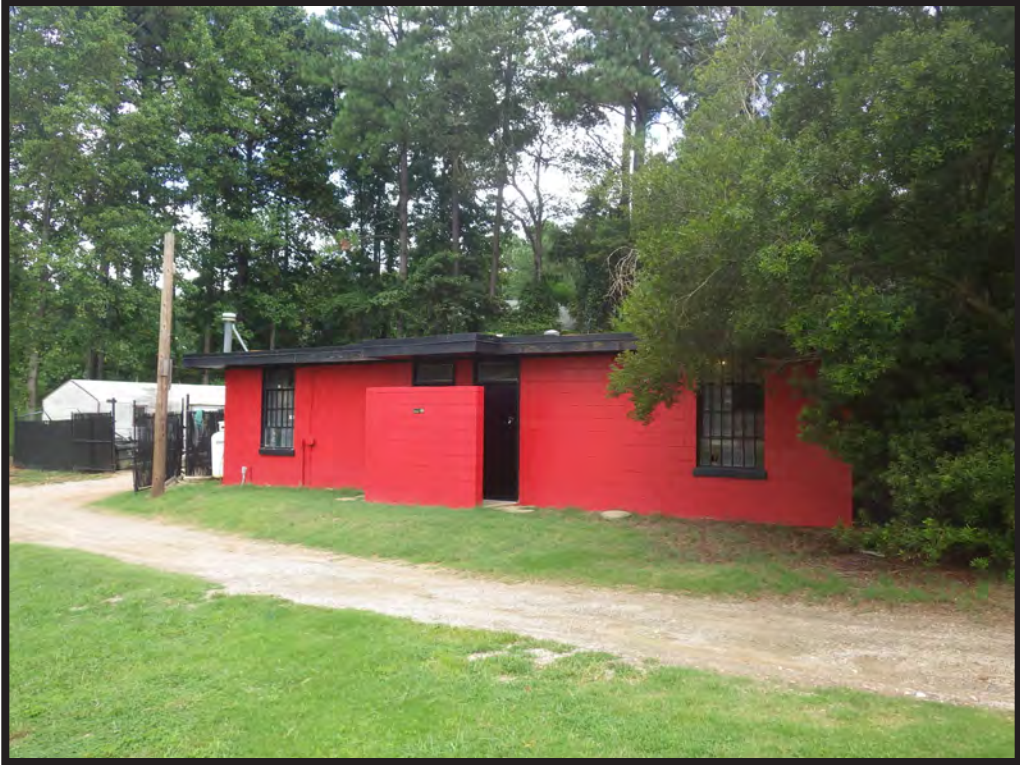
Figure 107. Maintenance Building, West Side
