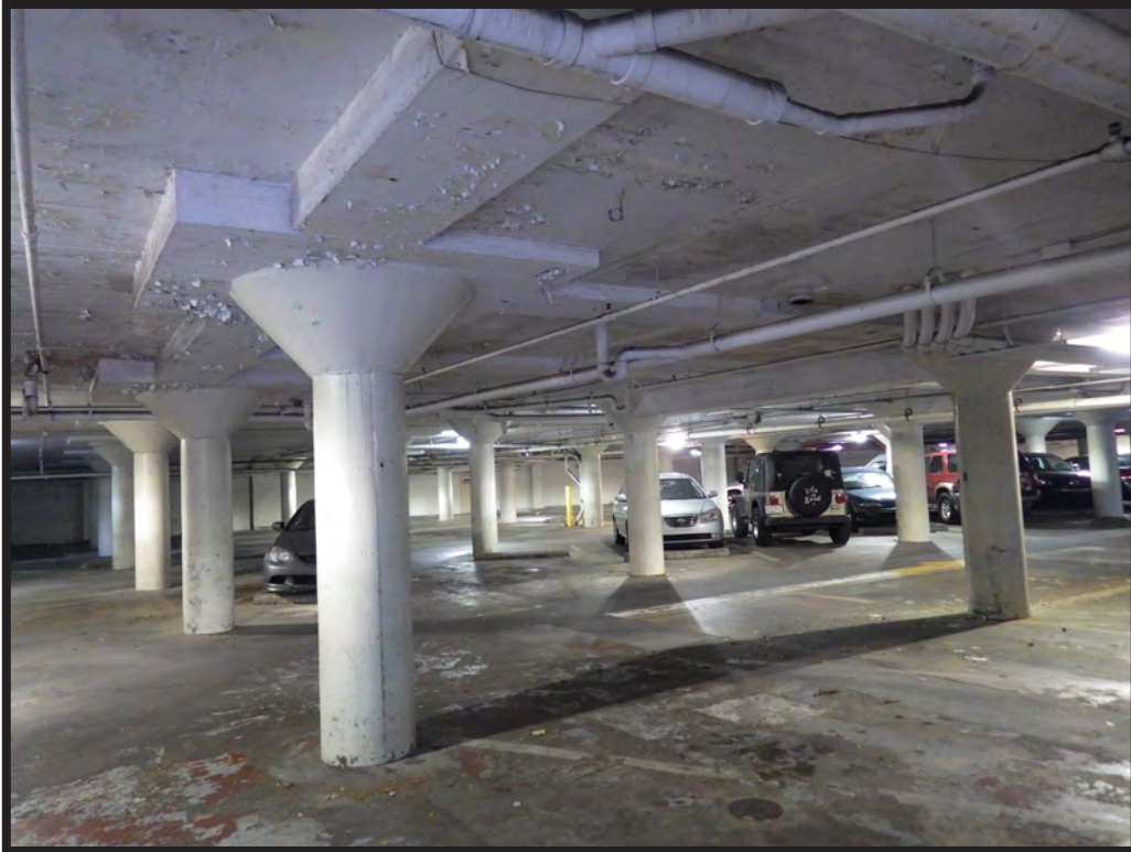
Figure 11. Royal Baking Company, Basement Supports
