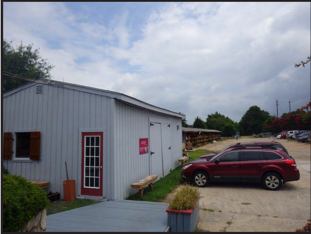
Figure 98. Storage Shed and Treated Lumber Shed
