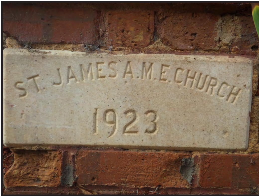
Figure 43. Cornerstone at Southeast Corner
